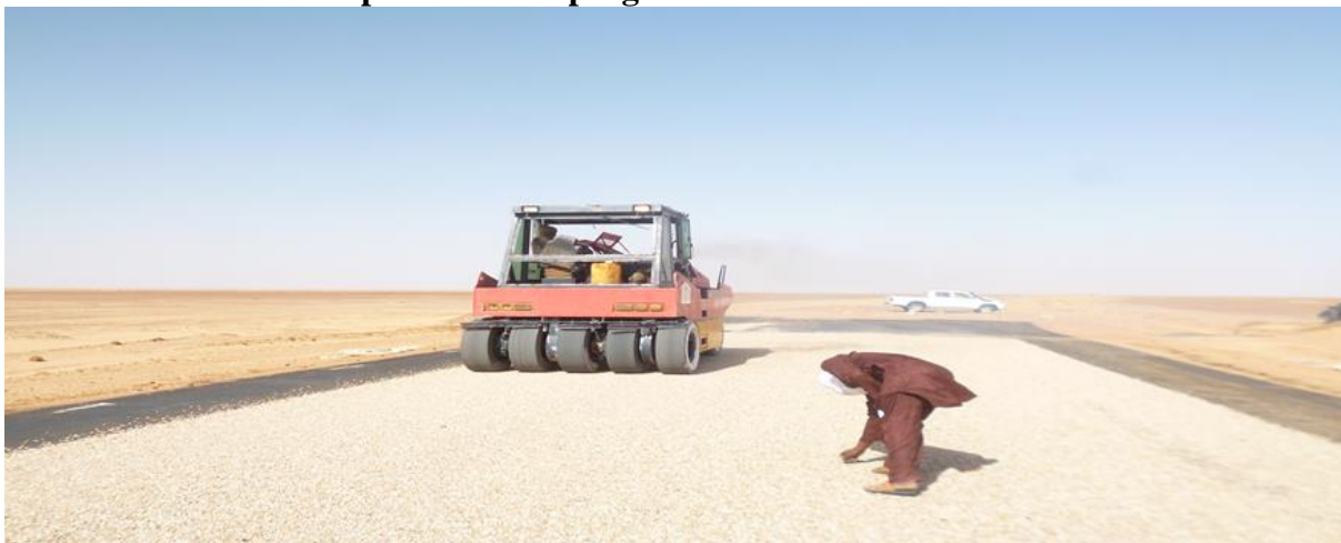
Chantier Route Arlit-Assamaka
